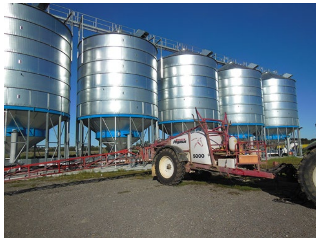
Capital expenditure on plant and infrastructure cannot be claimed as an operational expense to help minimise tax liabilities.
